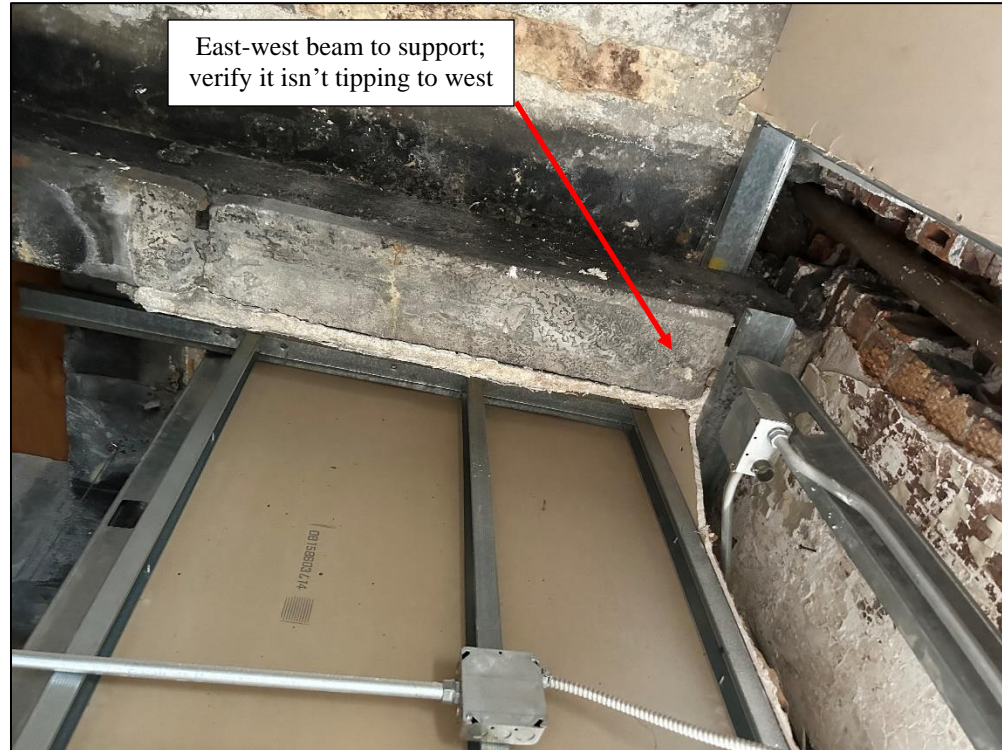
Photo 4 – Existing Beam to Support
