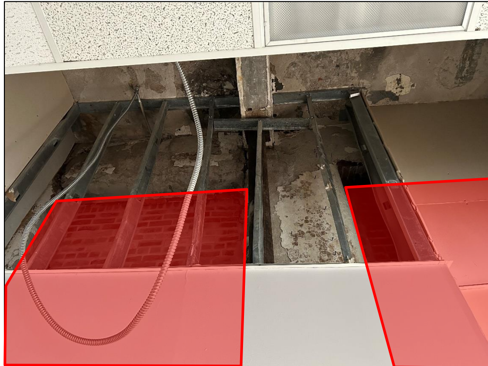
Photo 2 – Window Openings to Infill
